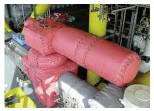
Darmatt <sup>™</sup> - a unique flexible, passive fire protection system that can meet 180 minutes blast protection up to 0.43 bar, protecting personnel and providing asset protection. DARMATT provides protection for valves, actuators, cable routes, conduits signal lines, junction boxes, solenoid stations, air receivers, process vessels and other equipment applications requiring fire protection.
