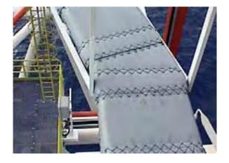
Darshield<sup>TM</sup> - rigid and compact engineered enclosures with up to 3 hrs of protection against flame temperatures in excess of  $1100^{\circ}$ C.
