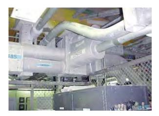
Darmatt KM1<sup>TM</sup> - is a fire protection barrier system developed for the protection of critical & safety electrical equipment in the nuclear & industrial markets.
